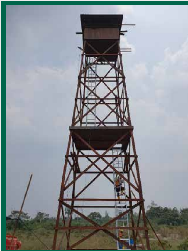
Observation tower Menara pengawas
